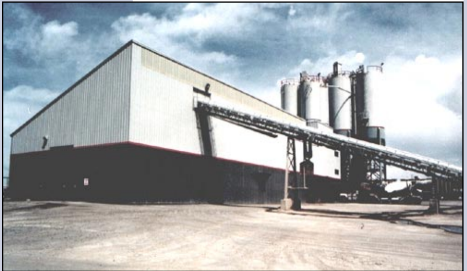
9.5 cubic yard Batch Plant
