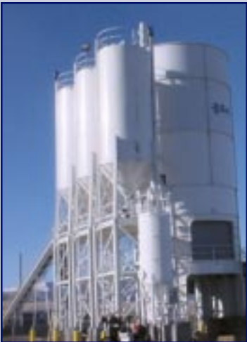
Six compartment aggregate storage bin - Transfer conveyor - Cement storage silo
